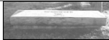
Burial vault slab Top of the concrete burial vault is left at grade forming an imitation ledger.
